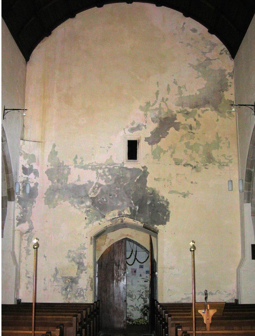
West wall damaged by water penetrating from the tower
