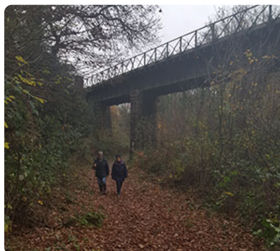
Footpath under railway viaduct in Luxulyan valley · Photo courtesy of Tabitha Stafford
