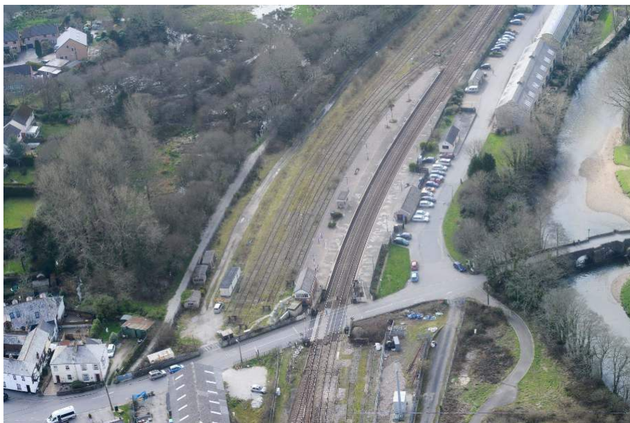
Figure 1: Ariel view of Lostwithiel station
