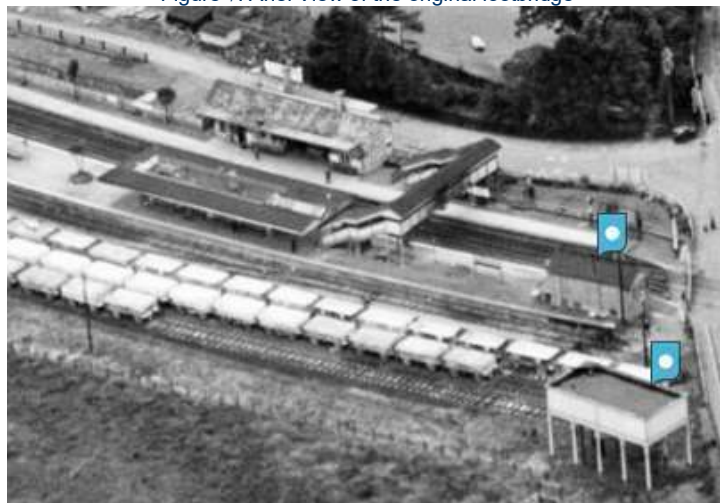
Figure 7: Ariel View of the original footbridge
