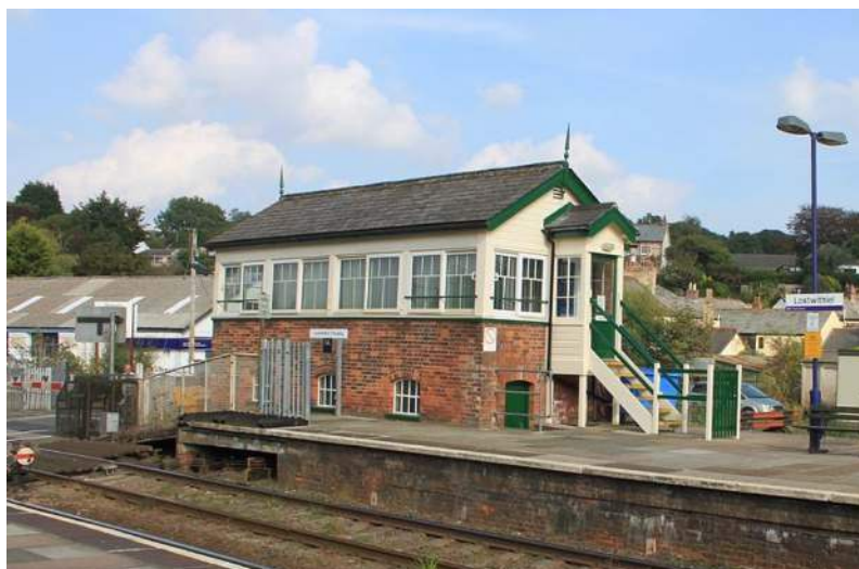
Figure 4 – Lostwithiel Signal Box, Grade II Listed
