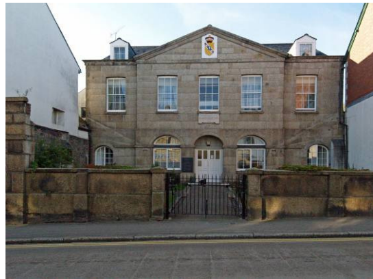
Old market house (1781), Queen Street, a granite ashlar frontage with a strong Palladian influence with central bays broken forward and surmounted by a triangular pediment. Note that only the façade survives; the remainder is a 20 th century rebuild
