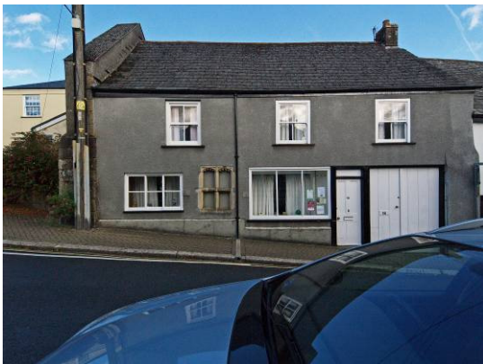
No 16 North Street, Lostwithiel: medieval window built into front wall of a 17 th century house
