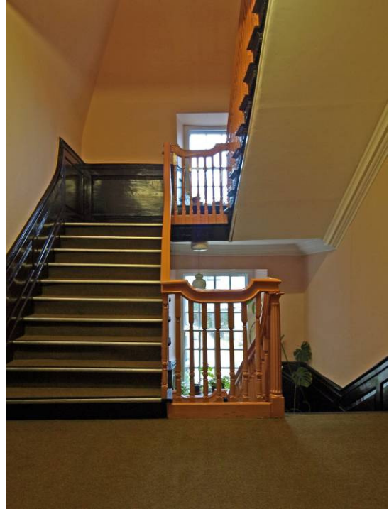
Edgcumbe House, Fore Street: fine mid 18 th century open-string staircase with column newels, turned balusters and ramped handrail, the stair wing lit by 18 th century sash windows with thick glazing bars. Edgcumbe house is an 18 th century rebuild of the frontage of a mansion house now called Taprell House
