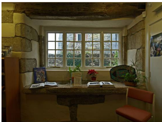
Window opening with granite sinks and moulded oak lintel
