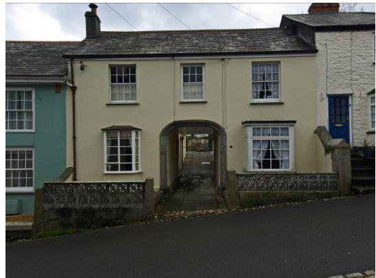
Nos. 4 and 5 Duke Street: moulded arched fragments reused to frame ope to former cottages at rear
