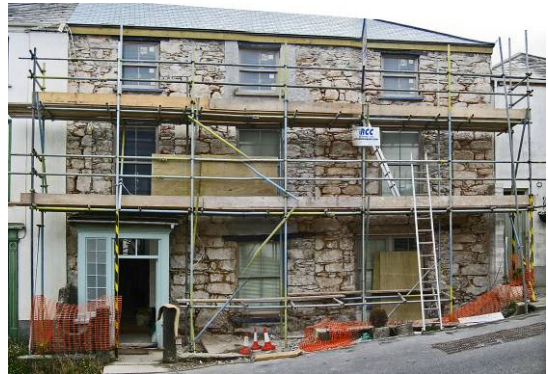
Avery House with stucco removed revealing earlier features
