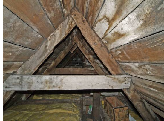
Former Debtors' Prison: 18 th century roof structure and lining of security boards
