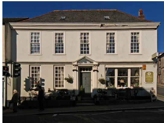
No. 8 Queen Street is a fine early 18 th century town house with original door-case and many original sash windows with thick glazing bars. The theme continues with a steep-pitched hipped roof over a moulded eaves cornice. A very unusual and rare feature in Cornwall is the mid-floor pseudo jetty with a moulded cornice
